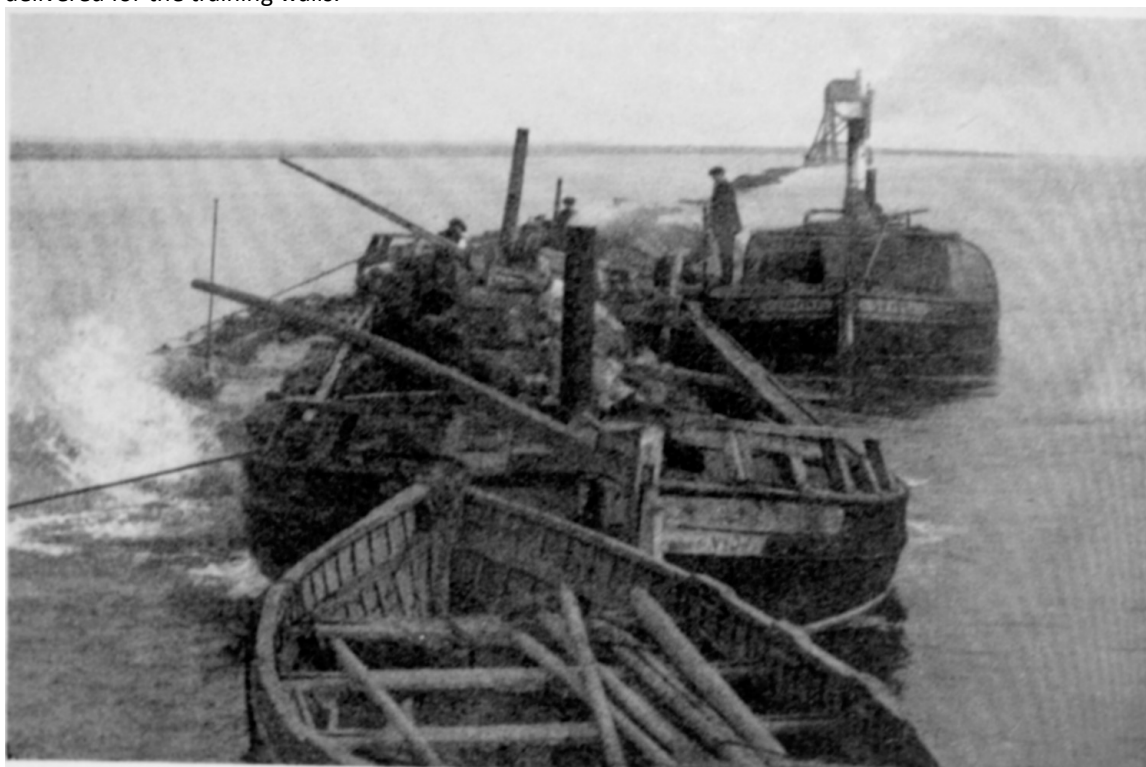
CANAL BARGES DISCHARGING STONE ON NORTH WALL AT 12½ MILE
